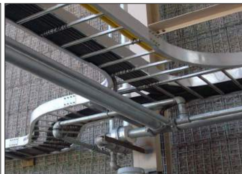
Cable Tray Installation
